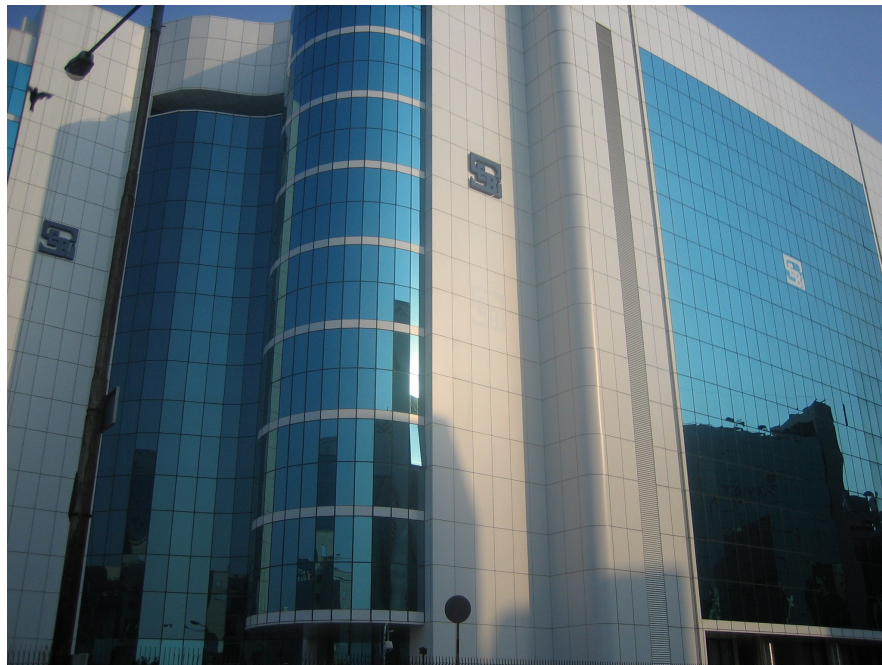
Sebi Building Mumbai.
